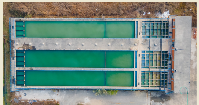
Manohara Water Treatment Plant
