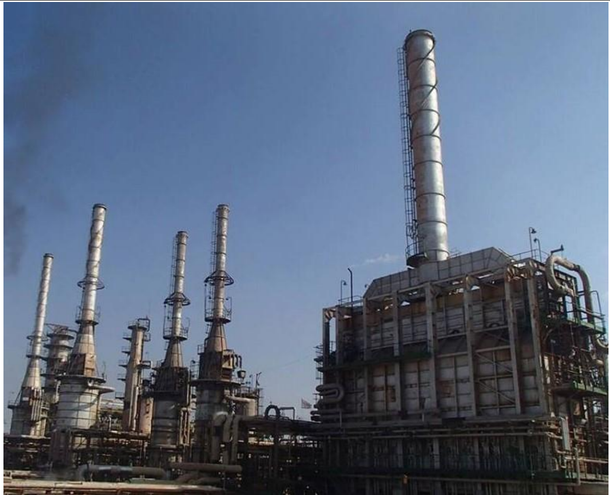
Existing plant of Basrah Refinery, next to which the new plant will be constructed under Basrah Refinery Upgrading Project funded by JICA's loans
