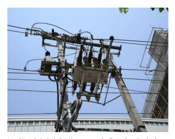
Load Break Switch (LBS) –automatically Isolate Faulted Sections of Electrical Distribution Systems at Bangalore District Upgradation Project
