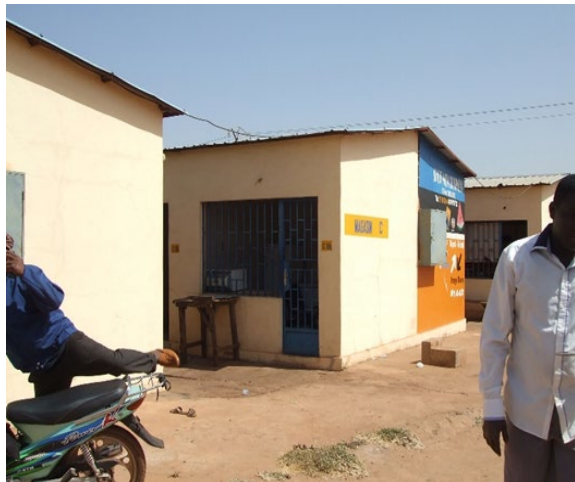
A kiosk for retailers distributing products other than fresh fish (constructed by AGMCPB (the management agency of MCPB) to revitalize the market)
