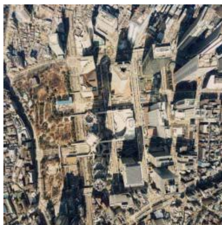
Slanting of buildings due to relative elevation differences (aerial photo example)
